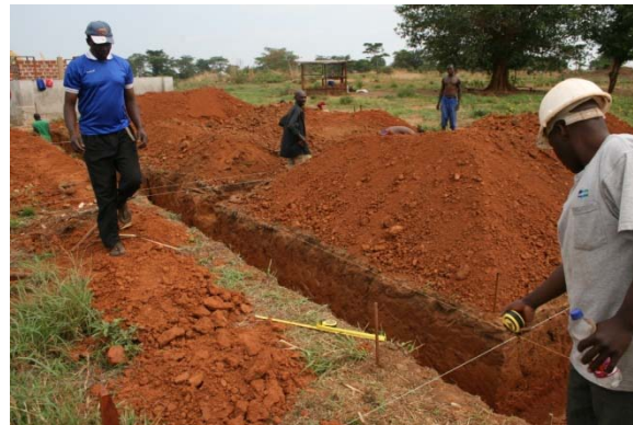
18 Boarding boys 2. Finished digging the foundation hole (↑).
