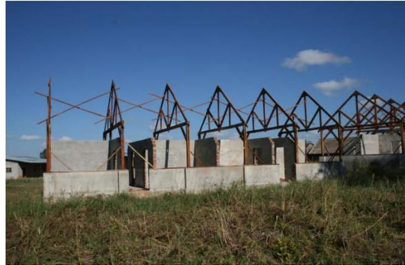
**18 Boarding Boys 2.** Finished plastering interior masonry and putting up the trussed rafters (↑).
