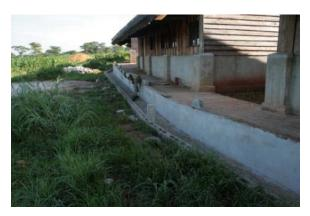
**Veranda.** On the girl's wing, at the back side of the veranda we finished pouring the concrete slab for the gutter, the single layer brick wall and plastering the veranda wall  $(\uparrow)$ .
