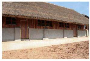
**9 Boarding Girls 2.** Finished covering the ventilation triangles, assembled and fixed all the doors (interior and exterior), fixed the window glasses ( $\uparrow$ ). Except for the floor, cable boxes, ceilings and painting this building is finished.
