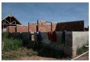
**17 Boarding Boys 1.** Finished ring beam interior masonry (个).
