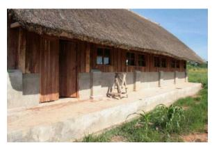
**11 Library 1.** Assembled and fixed the exterior doors front and back and fixed the window glasses. Finished door- and windowsills (↑). Except for the floor, cable boxes and painting this building is finished.
